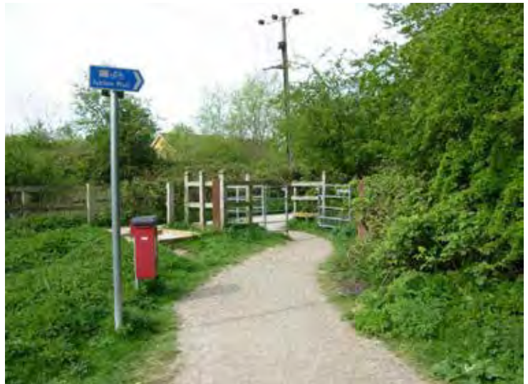
New surfacing and horse stile
